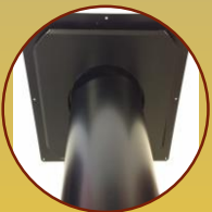
System 2 Firestop with Cover Plate
